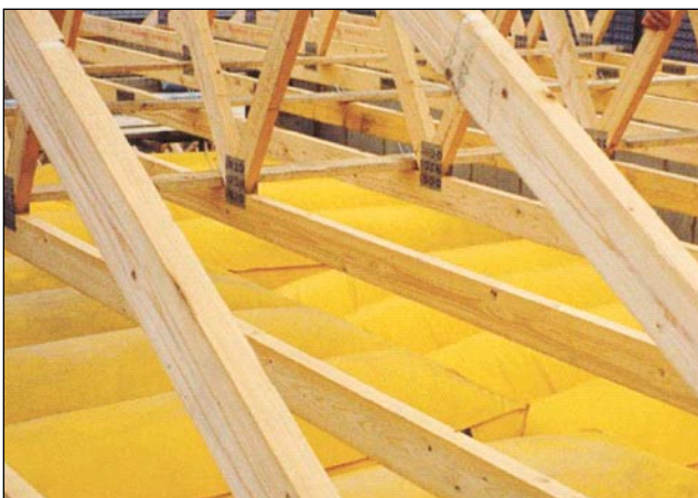
Figure 15(b) Air bags being used as a fall mitigation measure during roof work (Image courtesy of Airtek Safety Products Ltd)
