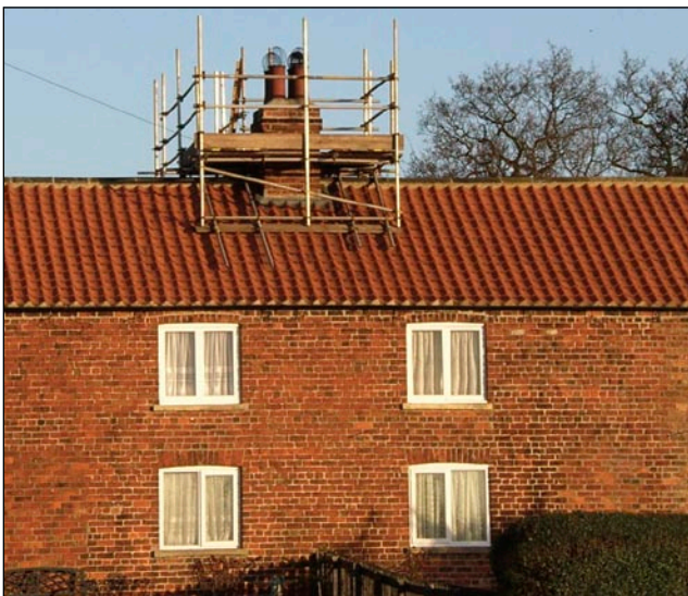
Figure 27 A traditional chimney scaffold
