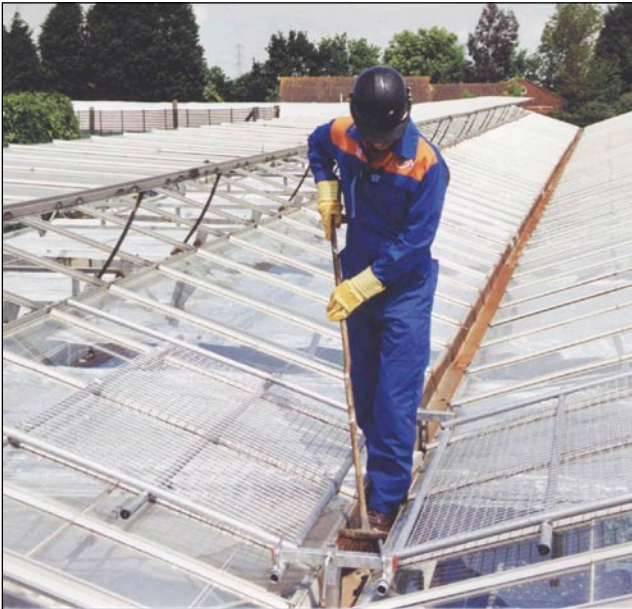
Figure 13 Valley walker used during gutter cleaning. This provides a protective mesh covering to either side of the operative, which moves progressively along the roof as the worker moves forward. The protective covering eliminates the risk of a fall through the fragile material (Image courtesy of Safesite Limited)
