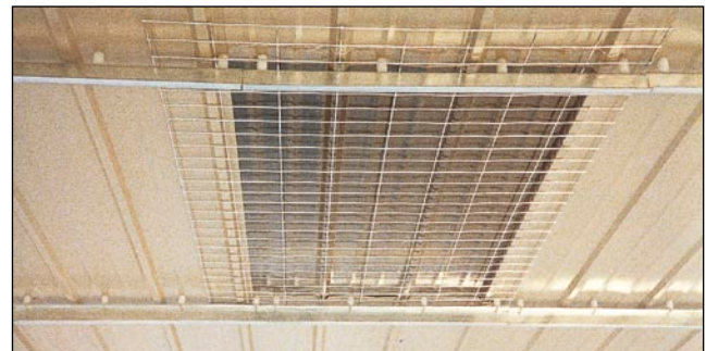
Figure 47 Galvanised mesh reinforcement between sheets of twin-skin roof light
