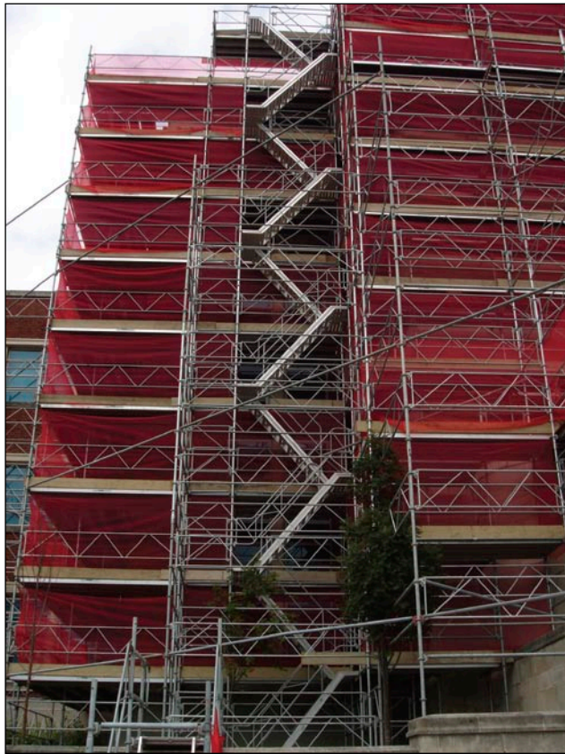
Figure 4 Stair towers provide good access. Make sure they are properly secured and erected (Image courtesy of Turner Access)
