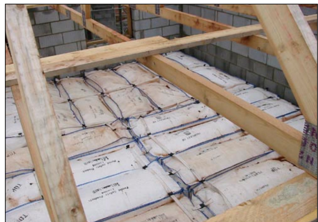
Figure 15(c) Bean bags being used as a fall mitigation measure during roofwork (Image courtesy of Forest Safety Products Ltd)
