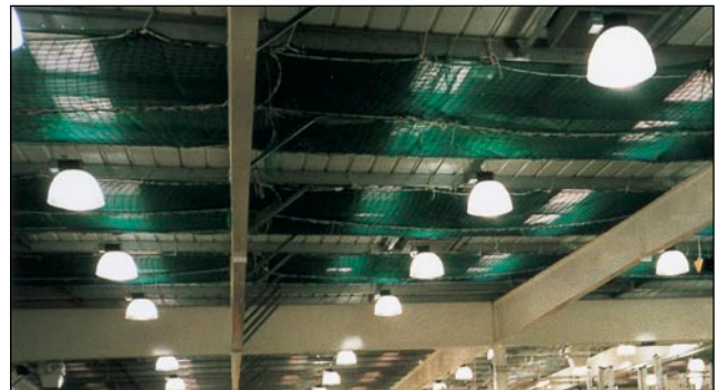
Figure 31 Safety netting used to provide protection for roof lights during minor roof works
