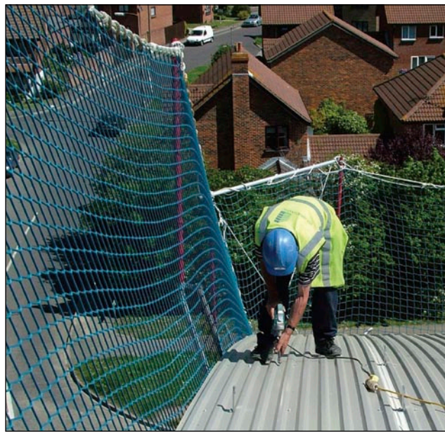
Figure 36 Net barrier system
